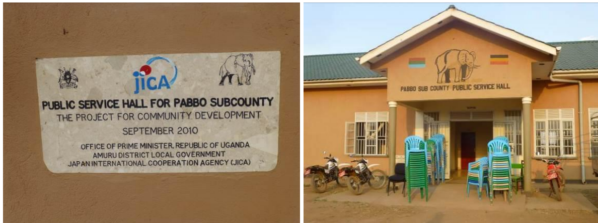
The completed Sub-county Hall in Pabbo Trading Centre, February 2013 (Photos: Ina Rehema Jahn)
